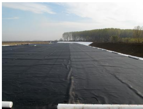
Photo 10. Application to new waste dumps
